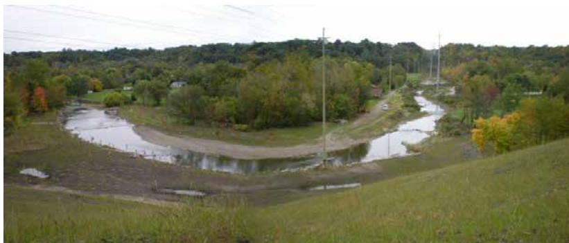
Relocated to its location in the 1970's, the stream moved more than 300' from its position at the beginning of the project (see below construction photo). Native floodplain vegetation including trees and whip plantings are beginning to establish.
