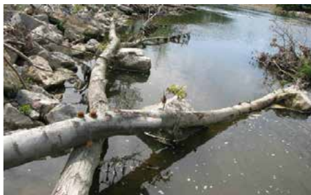
In stream log structures were imbedded into the shoreline to increase fish habitat, provide roughens in the stream, and armors channel.
