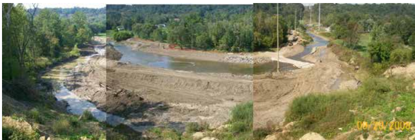
Relocated to its location in the 1970's, the stream moved more than 300' from its position at the beginning of the project (see below construction photo). Native floodplain vegetation including trees and whip plantings are beginning to establish.
